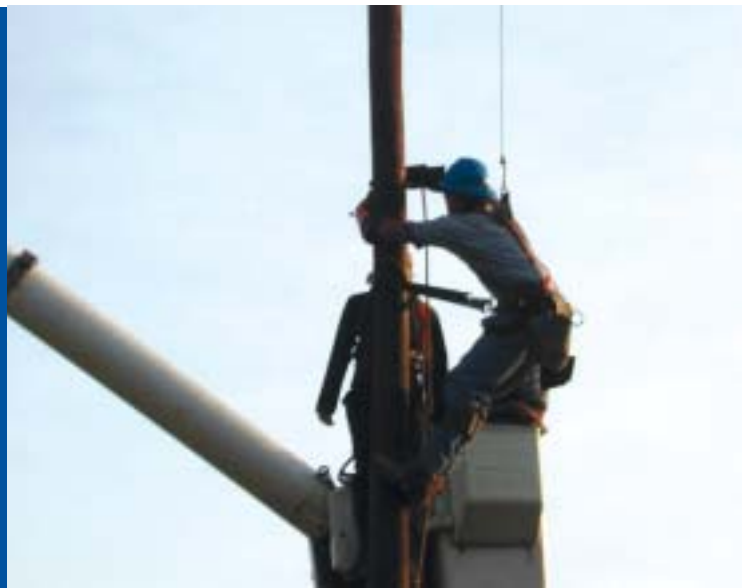
Randolph EMC linemen perform pole top rescue demonstration.
